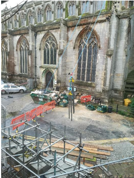
Scaffold poles coming down on a pulley system Long climb to get to work!
